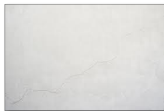
Hairline Cracks
